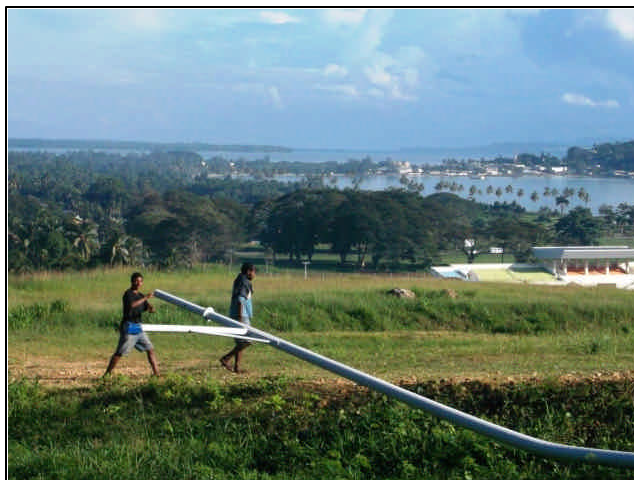
The bent lightpost hit by the van.
